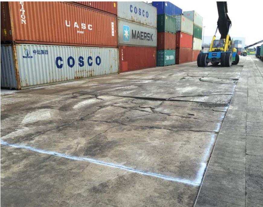
Area of damaged concrete marked out prior to removal.
