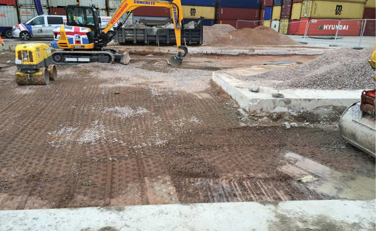
Slabs removed and stone compacted.
