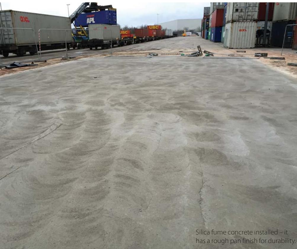
Silica fume concrete installed – it has a rough pan finish for durability.
